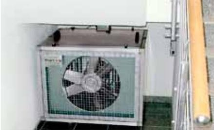
A fan module on the ground floor pressurises the stairwell in the event of fire.
